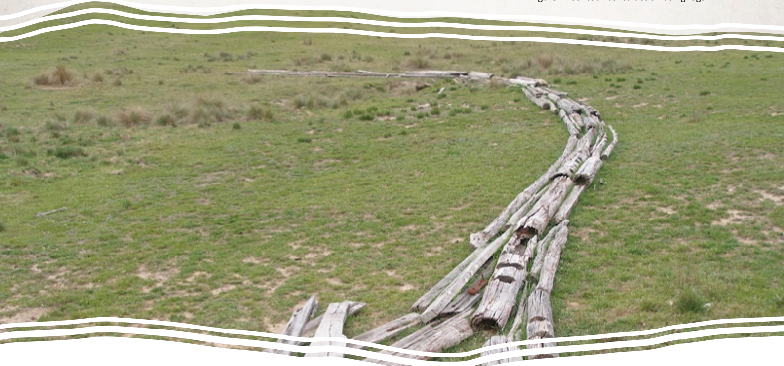
Figure 2: Contour construction using logs.
