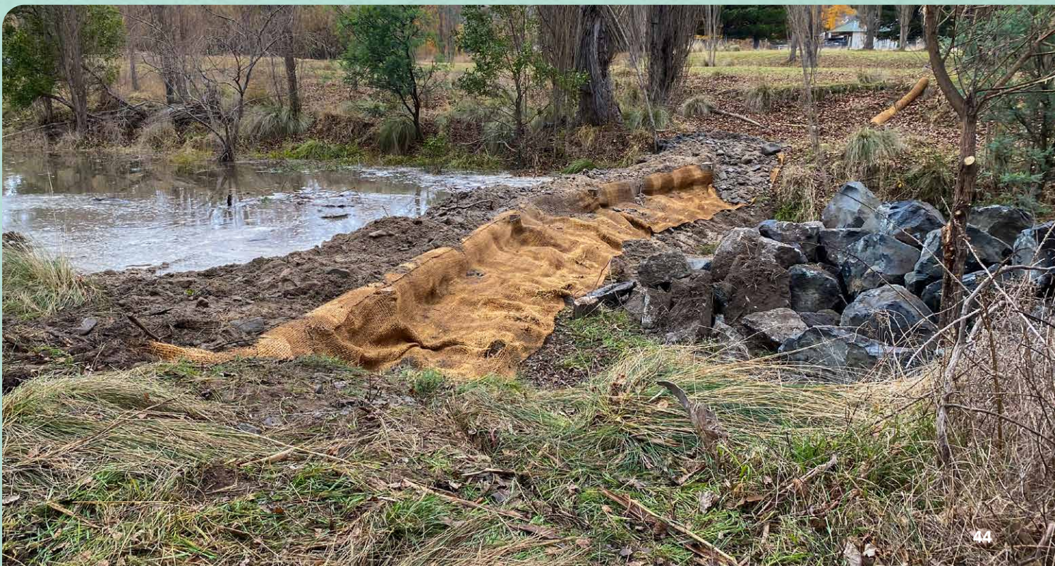
Figure 29: Geofabric in place on leaky weir installed at 'Tidbinbilla Station' ACT, 2023.
