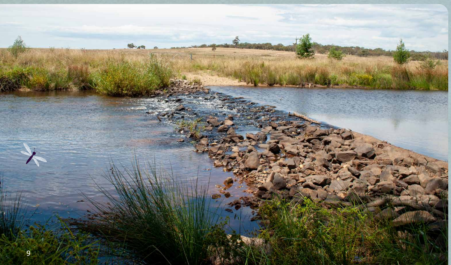
Figure 3: Landscape rehydration infrastructure (leaky weir) installed at ‘Palerang’, Mulloon NSW, 2022.
