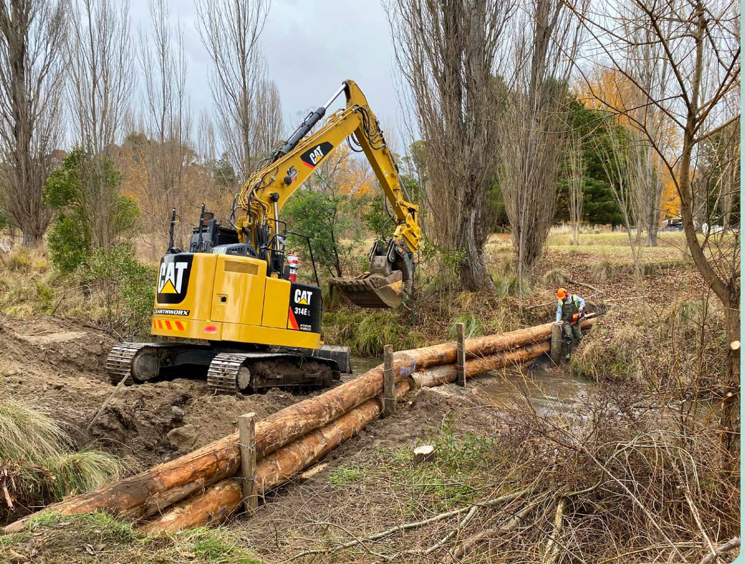
Figure 28: Hardwood logs securely fixed in leaky weir at 'Tidbinbilla Station' ACT, 2023.
