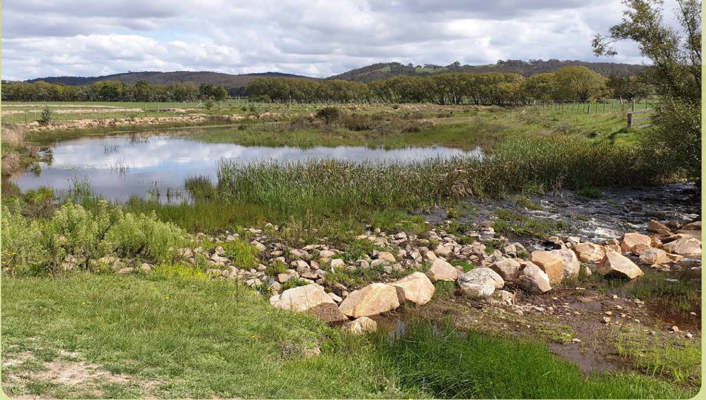
Figure 14: Landscape rehydration infrastructure (leaky weir) at 'Westview', Mulloon Creek NSW, 2020.
