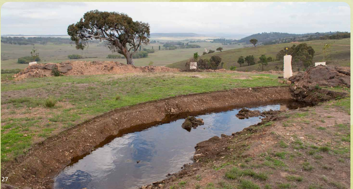
Figure 17: Top contour pond installed at 'Duralla', Mulloon Creek NSW, 2018.
