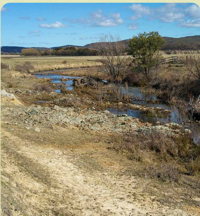
Figure 15: Landscape rehydration infrastructure (leaky weir) at 'Westview', Mulloon Creek NSW, 2015.
