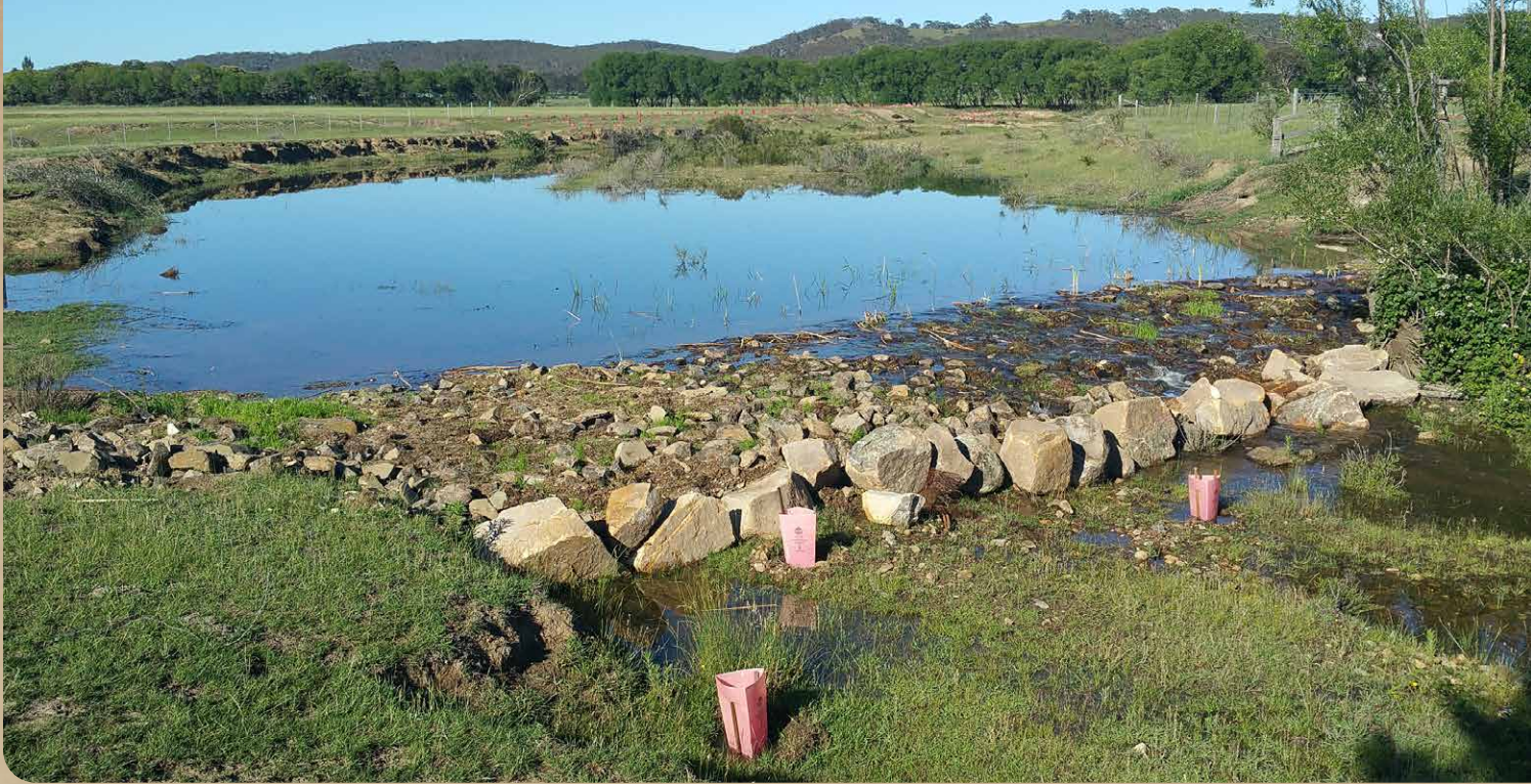
Figure 21: Log sill structure after construction at 'Westview', Mulloon NSW, December 2018.
