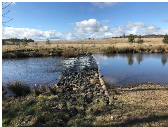
Figure 3: A “leaky weir” Mulloon Creek NSW
