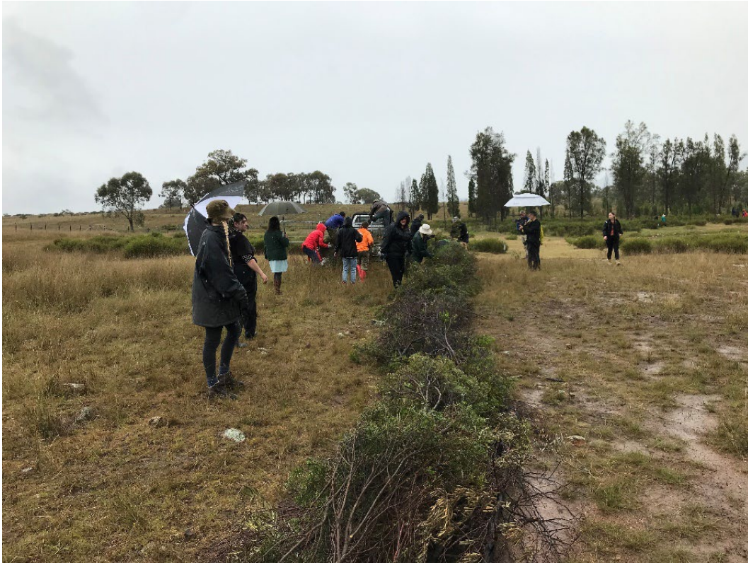
Figure 6: Brush-pack sieve erosion control on contour, Capertee Valley NSW
