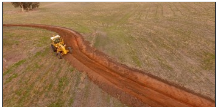
Above: Earth bank contours built at the Pensini's property 'Paraway' in May 2022..
