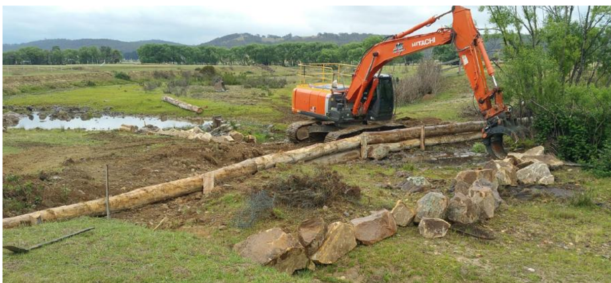
Figure 9 - leaky weir under construction at Westview farm (The Mulloon Institute, 2018)
