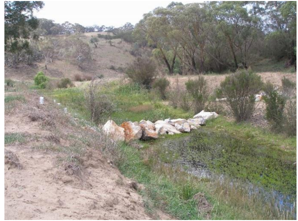
Figure B3: Example of an imported rock baffle in place on Mulloon Creek upstream of Westview.
