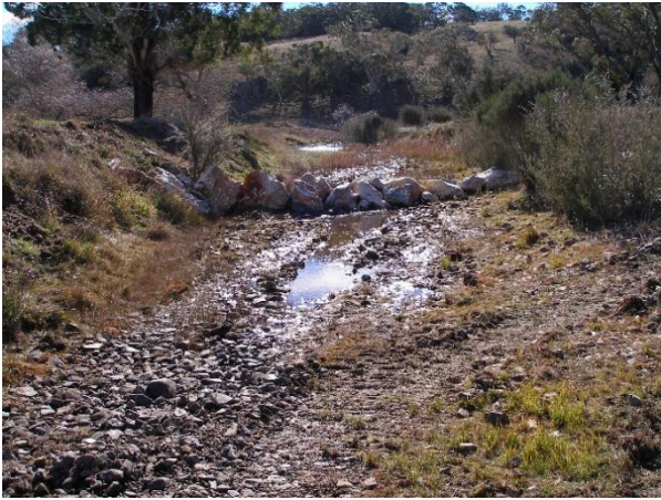
Figure B3: Example of an imported rock baffle in place on Mulloon Creek upstream of Westview.
