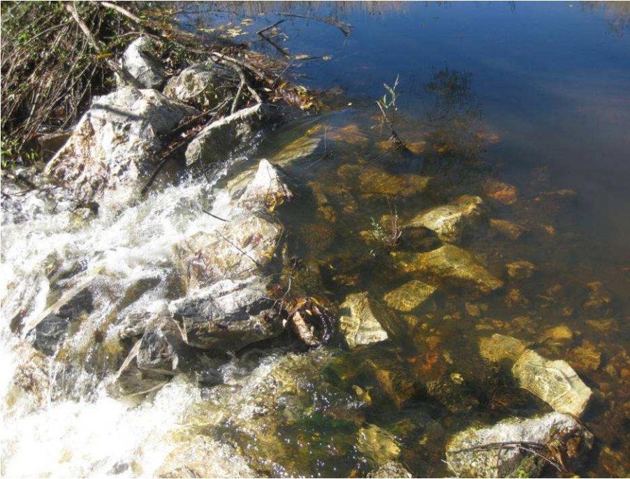
Figure 2.5. Leaky weir comprising rocks, mulch, sediment, plants and micro-organisms.
