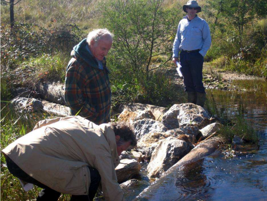
Figure 2.1. A log and limestone leaky weir at Mulloon Creek. L-R: Martin Royds (Chair, Natural Sequence Farming Association), Peter Andrews (Developer, Natural Sequence Farming) and Brad Davies (NSW Land and Property Management)
