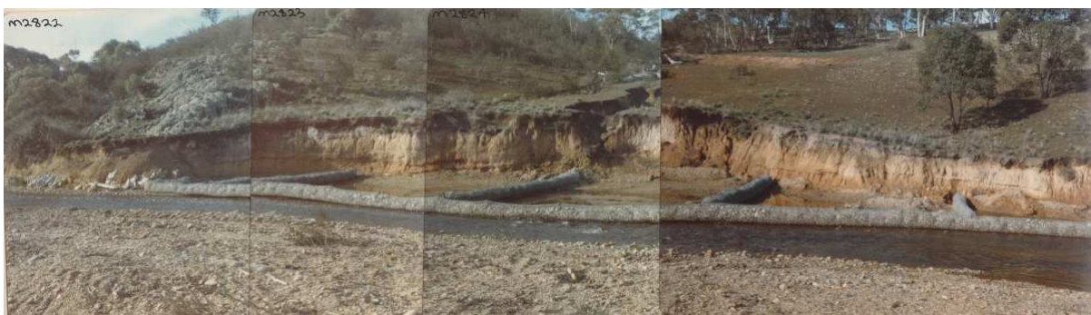
Figure 1.1. Rock sausages placed along Mulloon Creek in 1980 at the site where Weatherstation crossing is now located (see Table 2 and Figure 3 for location).
