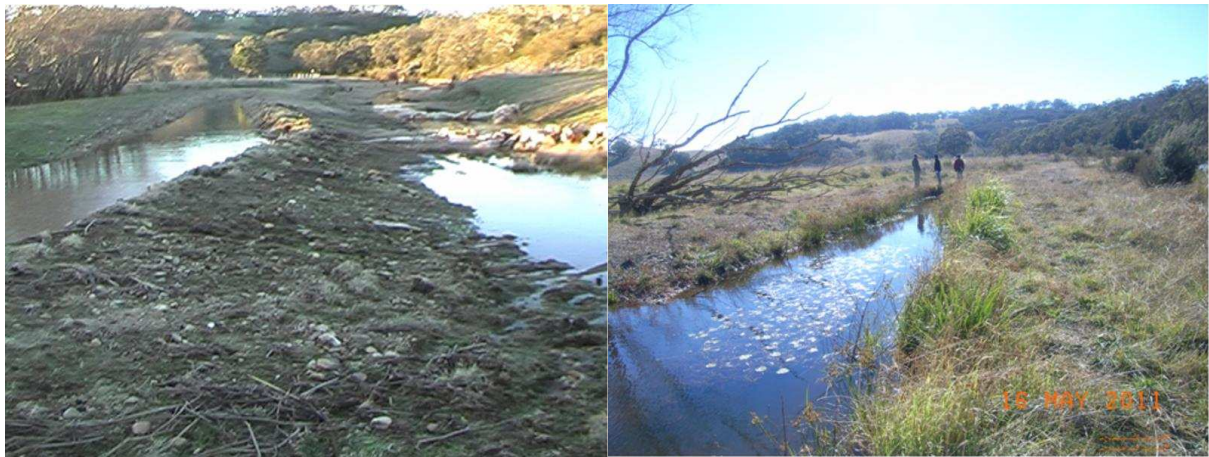
Figure 1.11. Downstream from Willows Crossing Complex (LW5b), Sept 2007 (left). Note rock sills to right of image in main channel. Also in May 2011 (right). Note the vegetation that has become well established in four years
