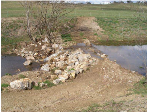
August 2007 following repairs and addition of rock
