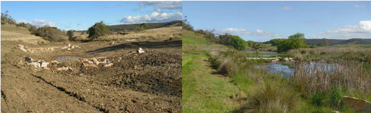
Figure 1.6. Triple Ponds Crossing (LW8) under construction 2006 on the left and Oct 2009 on the right.
