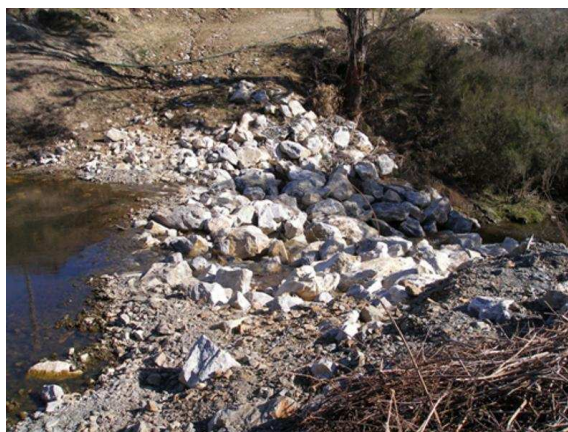
Figure 1.5. Pump-station Weir (LW14) in 2007.
