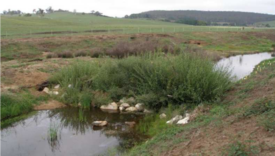
Figure 1.19. Mitchell's Weir showing the integration of vegetation with rocks that make up this structure.
