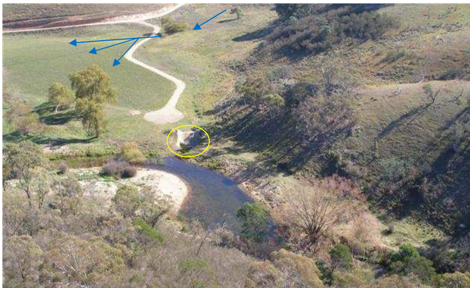
Figure 1.17. Photo from May 2007 showing recovery after reshaping. Water has been directed away from the flume (circled in yellow) onto the fan (new flow shown in blue arrows) and the incised channel has been reshaped. Note that a new track has been constructed that was not present in the previous Figure.
