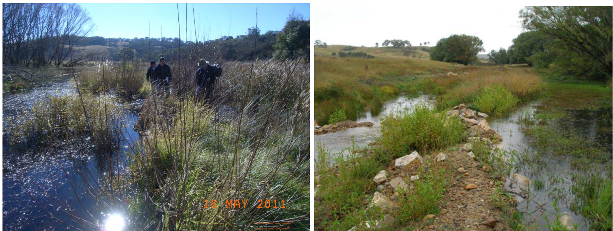
Figure 1.12. Downstream of Willows Crossing Complex (LW5b) at the upstream limit of the structure (left). Note extensive aquatic vegetation growing in main channel on RHS of image. Right photo - Downstream of Willows Crossing Complex (LW5b). Rocks were used to repair some flood damage creating an additional rock sill.
