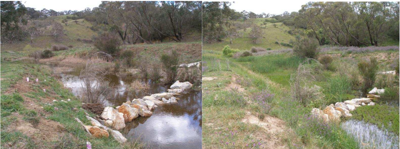
Figure 1.9. Rock sill downstream of Weather Station Crossing (LW3) Jun 2007 (left) and Aug 2008 (right).
