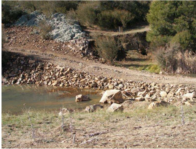
Figure 1.10. Weather Station Crossing (LW4) June 2006, this rock sill was constructed on a natural rock bar.
