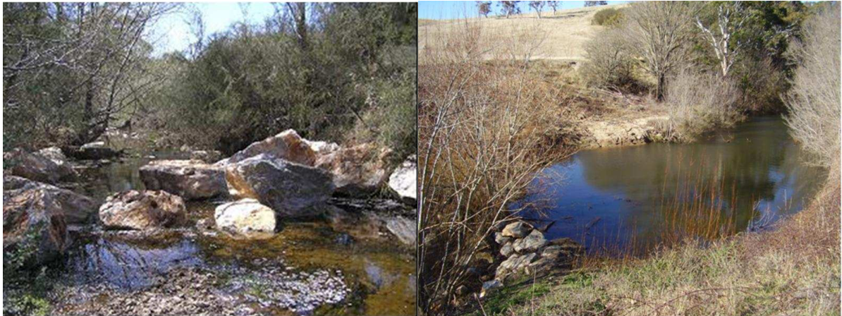
Figure 1.14 'Goldneys Gate' (LW1) (left) is a baffled structure which attenuates river flow. Willy's Ripl (LW13) (right) is a naturally occurring rock bar that was augmented with rock creating an extensive pool
