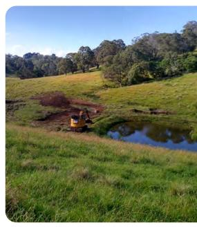
Incorporating existing infrastructure into landscape rehydration works, with ponds and sills added to retain water runoff from current dam.
